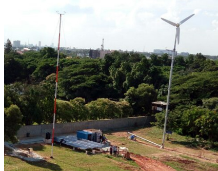
Fig.23 10 kW WiSH system at Renewable Energy Farm, Kodihalli Campus.
