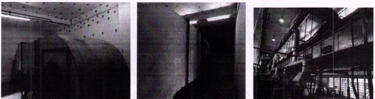
Fig.4 Blowers and HVAC ducting in the process area with louvres also shown
